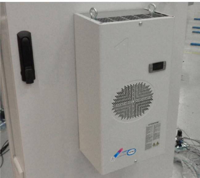
Air conditioner to be used in areas where the temperature exceeds xxx °C. Cooling capacity 640W. ???
