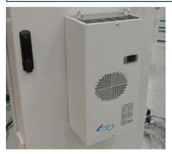
Air conditioner to be used in areas where the temperature exceeds xxx  $^{\circ}$ C. Cooling capacity 640W. ???
